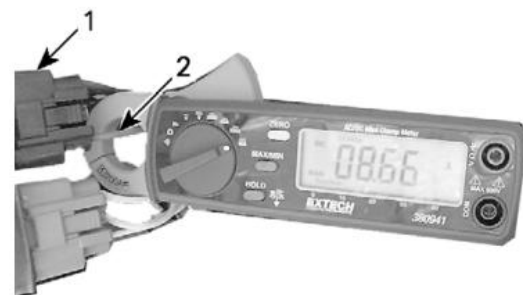
DC CURRENT TEST WITH INDUCTIVE AMMETER 1. Output connector of voltage regulator 2. Ammeter clamped over RED wire
